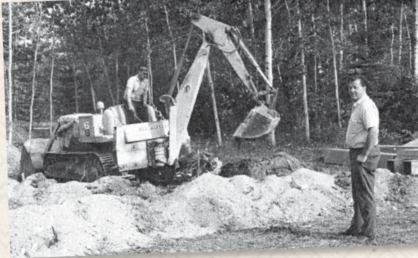
Alex Rawluk, Chairman of the Gypsumville School District Board, checks on the progress being made in the installation of the mobile living units for teachers in Gypsumville. The Department of Youth and Education spent about $40,000 during the summer to improve school facilities and teachers' living quarters in the town. The move followed the release of the highly critical Society report on education facilities last June.
